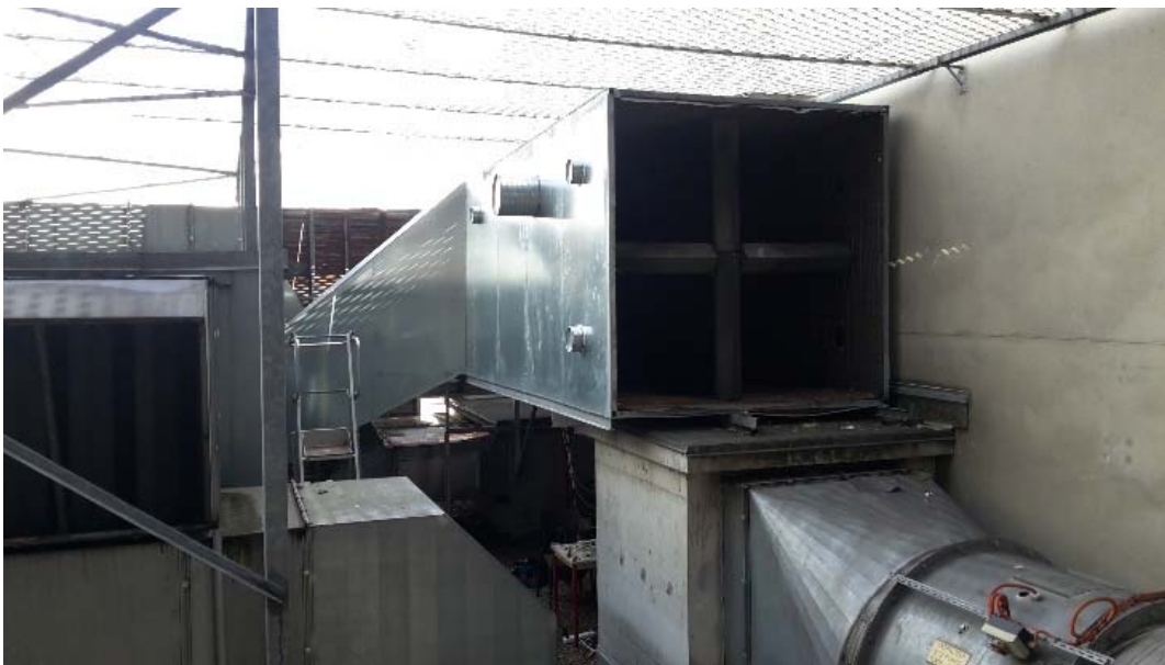
Installation EolAc chantier DARTY TERNES
